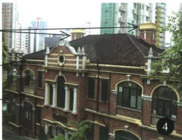
Chimneys Cornice String Course
